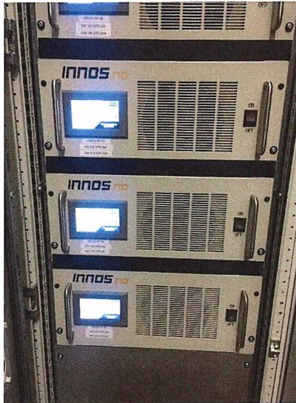
Figure 2: Weight Watcher Reverse Current Control Unit
